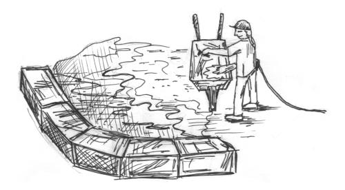
Letting any materials enter the stormwater system may result in fines
