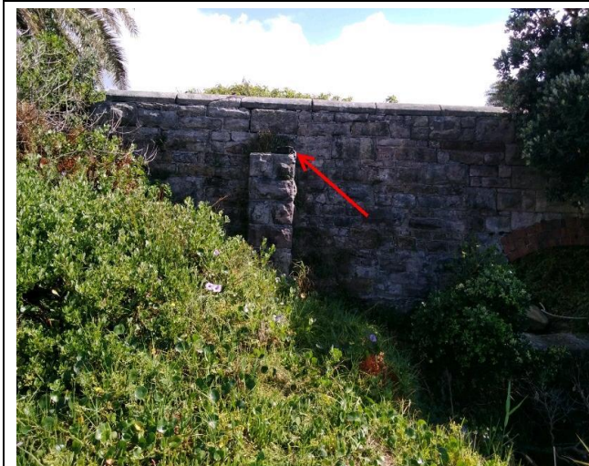
Location: Northern elevation, on stone retaining wall Result: <0.01 f/ml Image Id: 230320-121154
