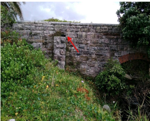
Location: Northern elevation, on stone retaining wall Result: <0.01 f/ml Image Id: 230228-095933
