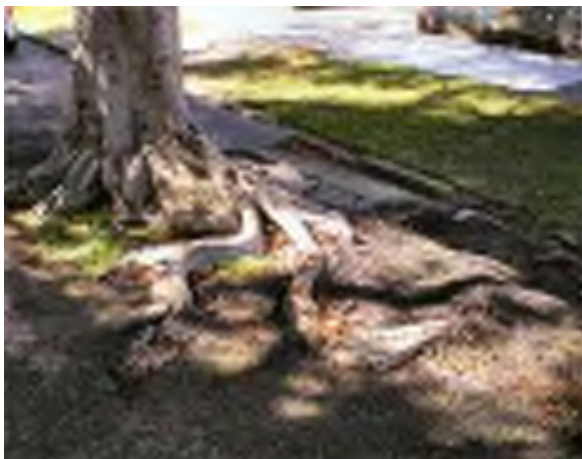
Photo 6: Existing kerb and guttering within Duke Street area is affected by tree roots.
