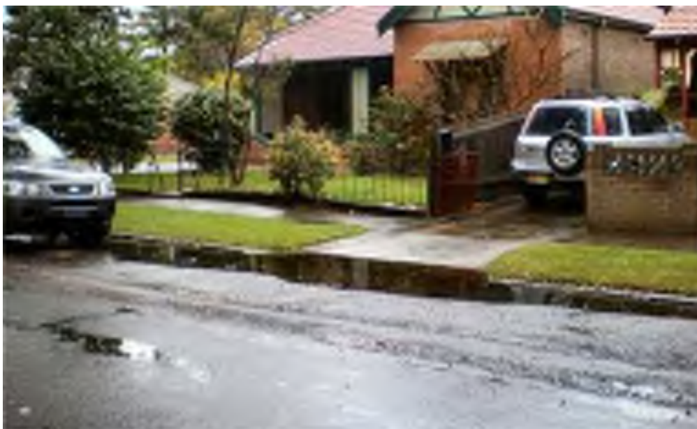
Photo 8: Ponding in front of Duke Street property access following minor rainfall.
