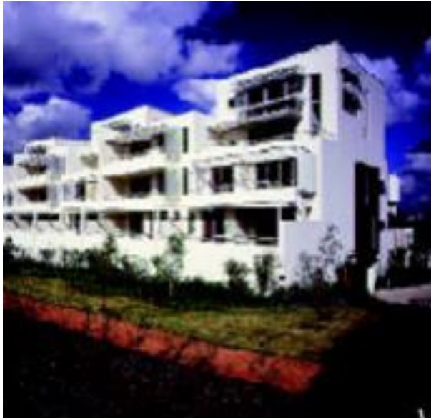
Figure 75: Sun shading is an integral component of the building form and facade design.
