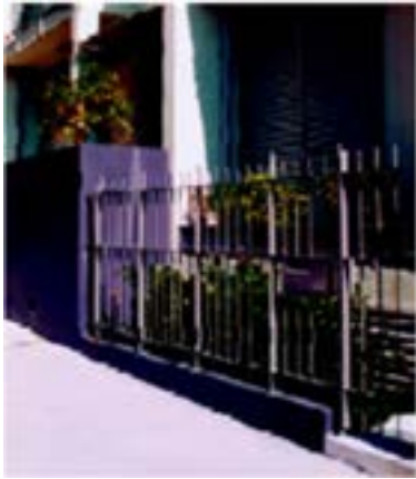
Figure 70: Street level picket fencing with planting provides screening to car park ventilation louvres
