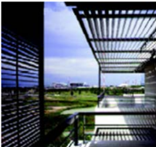
Figure 74: A combination of louvres provides shading for different times of the day.
