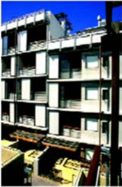
Figure 60: Building elements provide privacy between spaces: pergolas limit overlooking, solid walls and sliding screens limit horizontal views.
