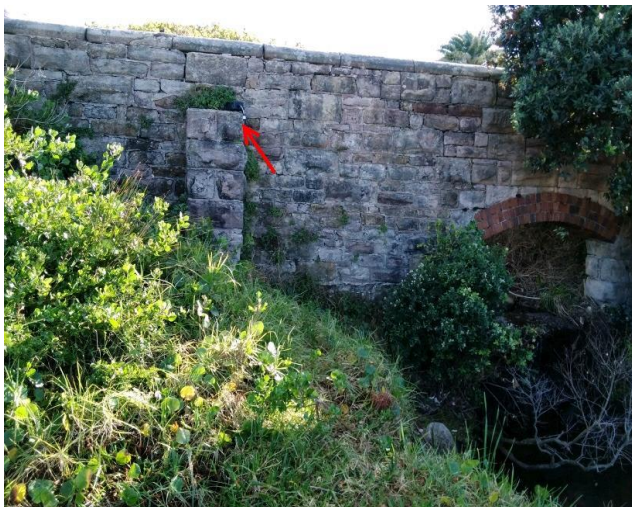
Location: Northern elevation, on stone retaining wall Result: <0.01 f/ml Image Id: 230703-093445
