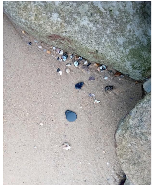
Notes: Visual surface clearance inspection following removal of suspected asbestos containing fragment
