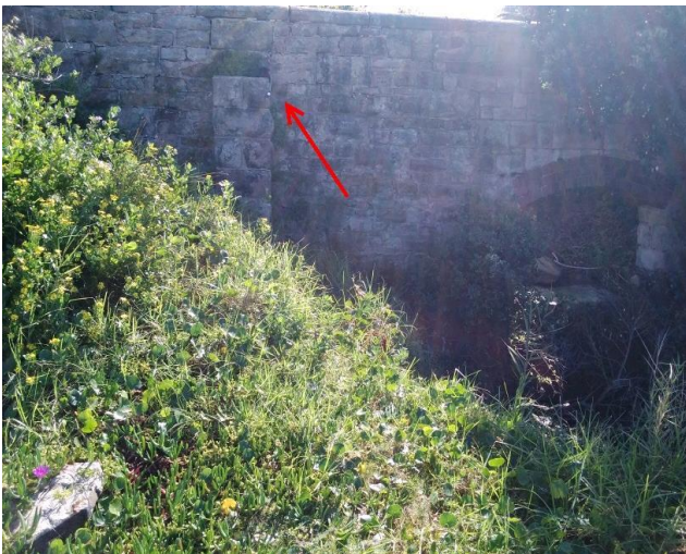
Location: Northern elevation, on stone retaining wall Result: <0.01 f/ml Image Id: 230523-115110
