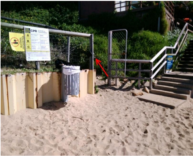
Location: Western elevation, Beach entry, on fence Result: <0.01 f/ml Image Id: 230523-115035
