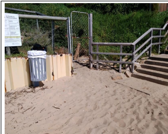
Location: Western elevation, Beach entry, on fence Result: <0.01 f/ml Image Id: 230310-102533
