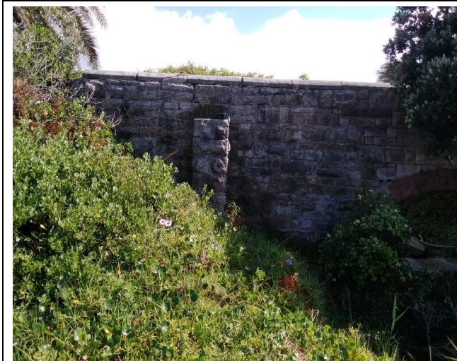
Location: Northern elevation, on stone retaining wall Result: <0.01 f/ml Image Id: 230310-103557
