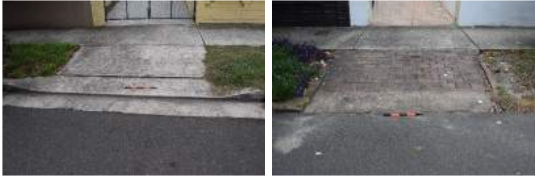
Figure 5: Two forms of driveways, featuring concrete (left) and brick pavers with concrete lowered kerb (right). If the image on the left, the kerbs either side of the driveway are of concrete while the image of the right shows kerbs of sandstone.
