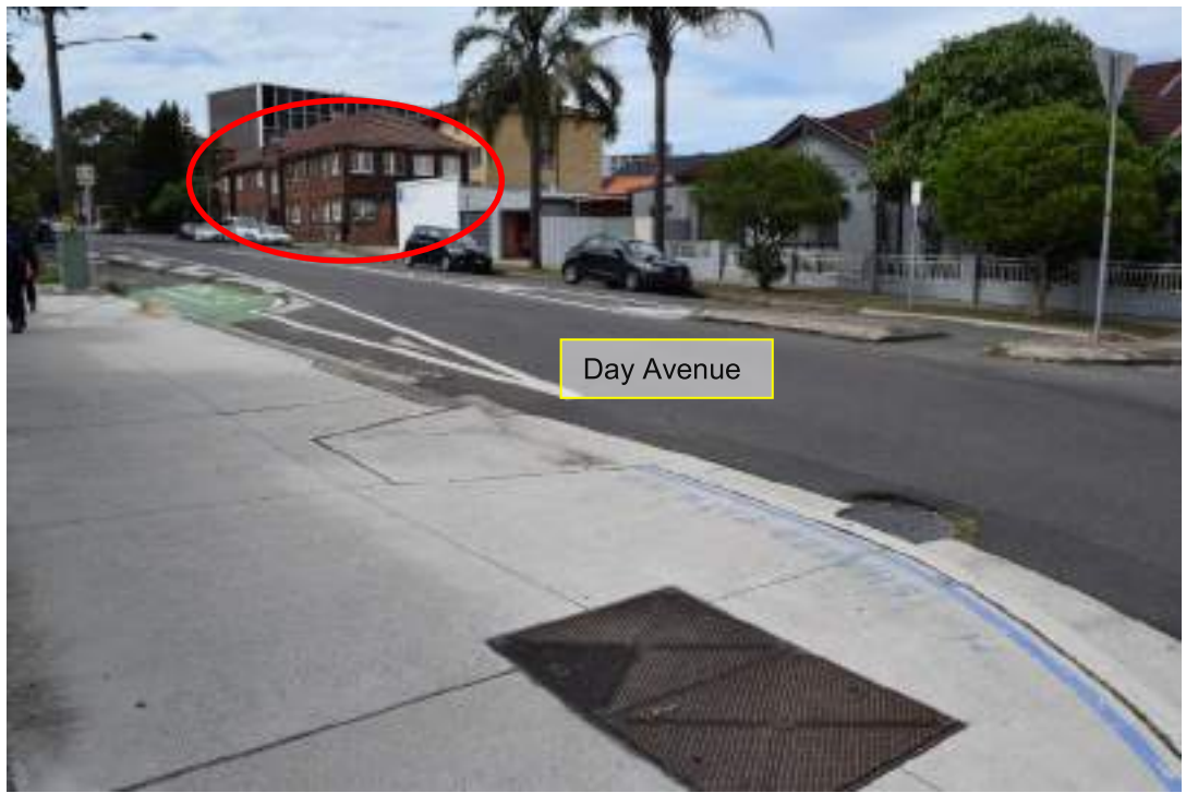
Figure 7: Looking east along Day Avenue from the intersection with Doncaster Avenue, with the separated cycleway on the left and an Inter-War apartment (circled in red) located in the background.
