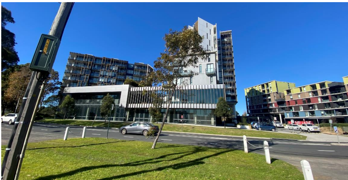
Figure 21 No. 132-136 Epsom Road as viewed from Link Road
