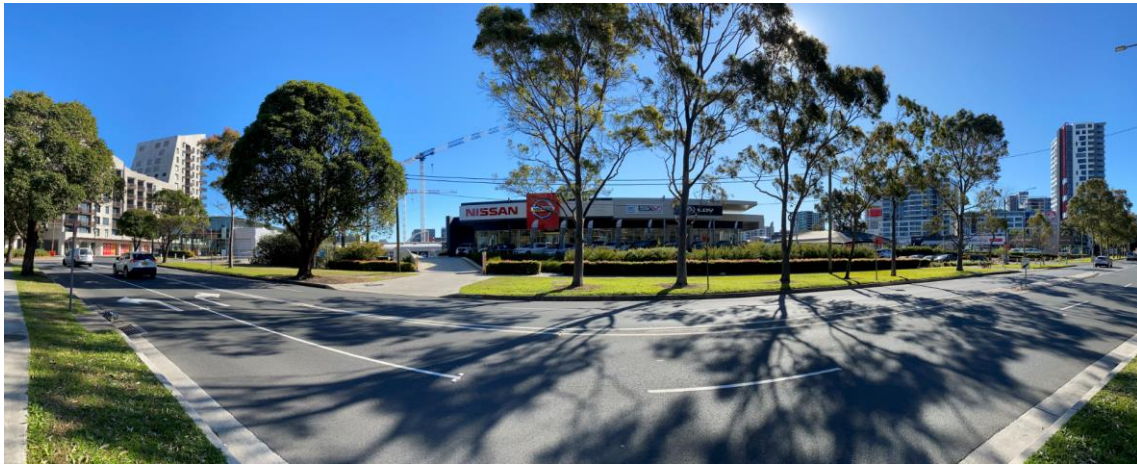
Figure 4 Subject site as viewed from Link Road
