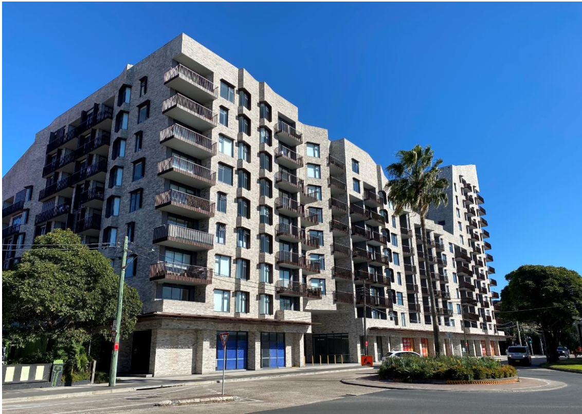
Figure 22 No. 67 Epsom Road as viewed from Link Road
