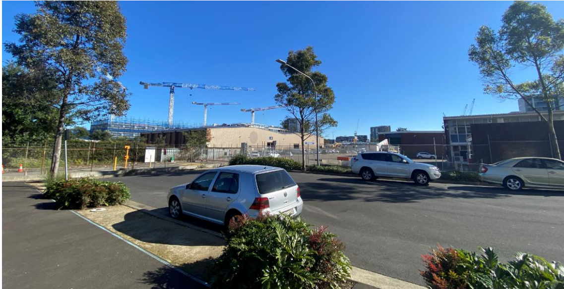
Figure 18 No. 130 Joynton Avenue as viewed from Defries Avenue
