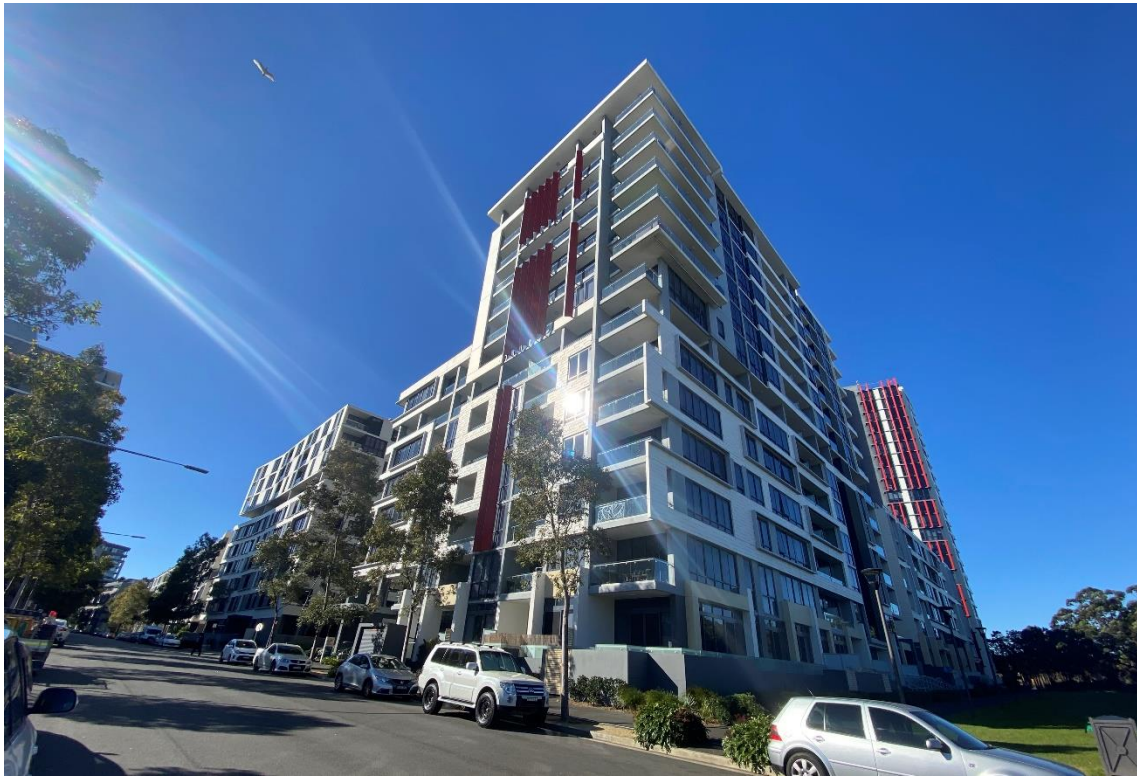
Figure 16 Developments to the north and north-east as viewed from Defries Avenue
