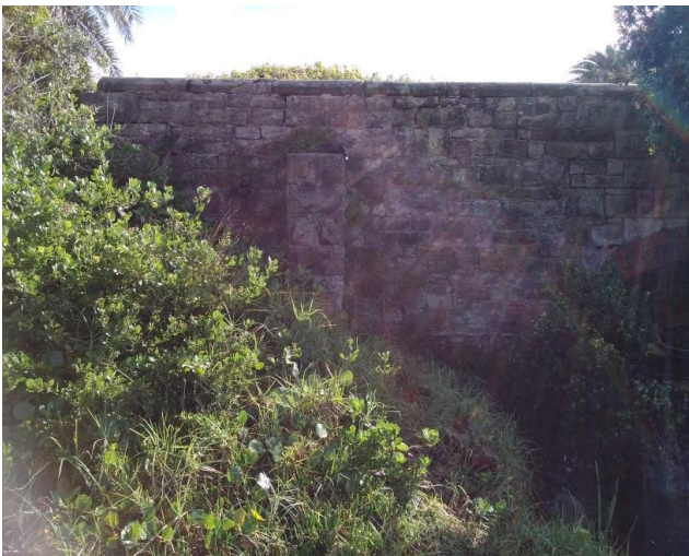
Location: Northern elevation, on stone retaining wall Result: <0.01 f/ml Image Id: 230613-102944
