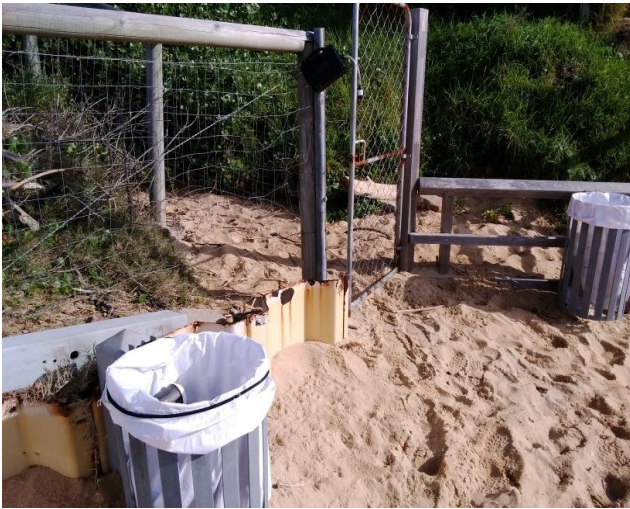
Location: Western elevation, Beach entry, on fence Result: <0.01 f/ml Image Id: 230613-102205
