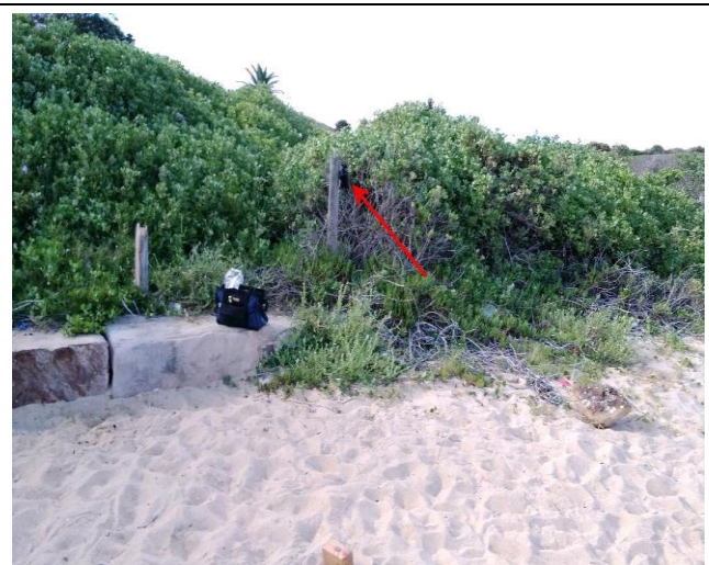
Location: Southern elevation, on pole Result: <0.01 f/ml Image Id: 230129-180643
