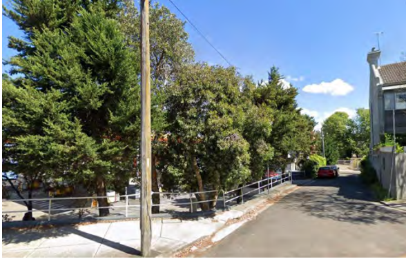
Photo 7: Intersection of William Lane & Betty Lane, retaining wall to manage topography
