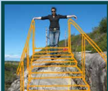
Steel access stairs provide safe access to the top of the sandstone escarpment with spectacular views.
