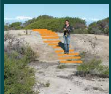
Minor access stairs and stepped boardwalks provide safe access over rock ledges and steep grade changes.
