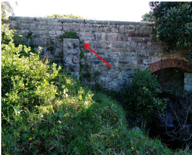
Location: Northern elevation, on stone retaining wall Result: <0.01 f/ml Image Id: 230610-094840
