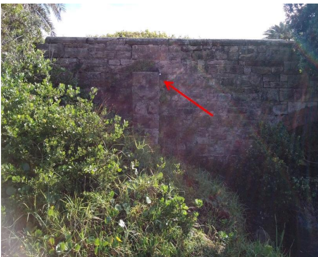
Location: Northern elevation, on stone retaining wall Result: <0.01 f/ml Image Id: 230617-102553
