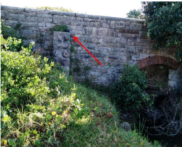
Location: Northern elevation, on stone retaining wall Result: <0.01 f/ml Image Id: 230711-102553
