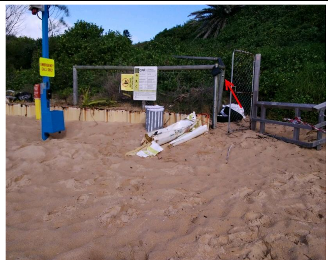
Location: Western elevation, Beach entry, on fence Result: <0.01 f/ml Image Id: 230517-100906
