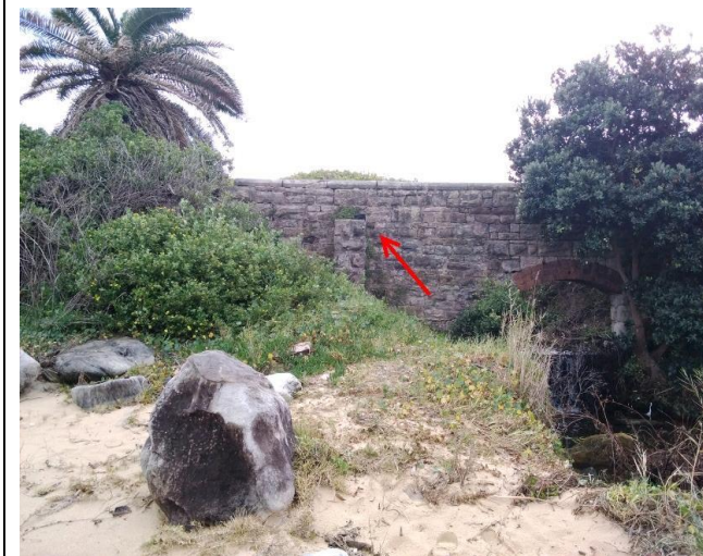
Location: Northern elevation, on stone retaining wall Result: <0.01 f/ml Image Id: 230517-101257
