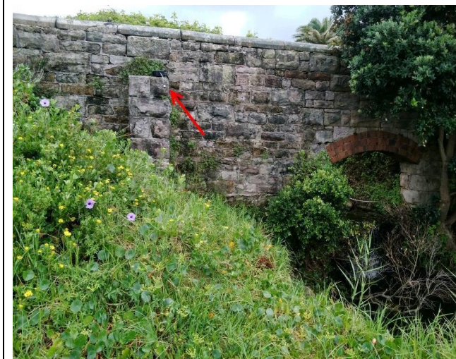
Location: Northern elevation, on stone retaining wall Result: <0.01 f/ml Image Id: 230406-092949
