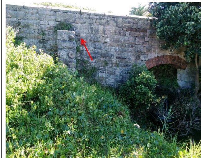
Location: Northern elevation, on stone retaining wall Result: <0.01 f/ml Image Id: 230330-101830
