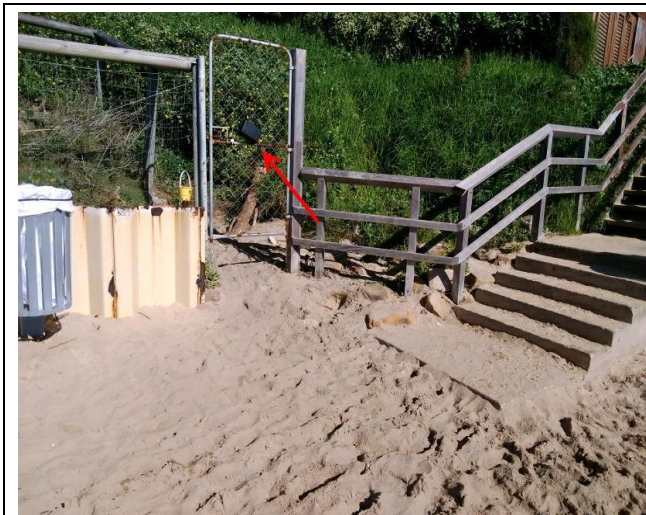
Location: Western elevation, Beach entry, on fence Result: <0.01 f/ml Image Id: 230330-100942
