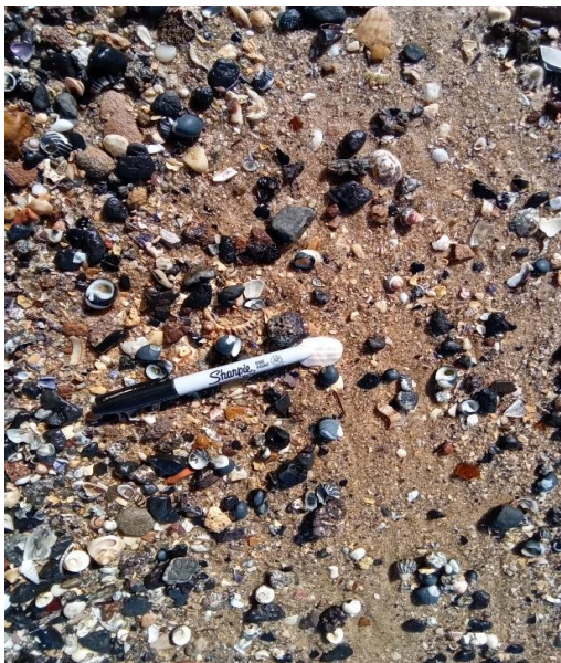
Notes: Visual clearance inspection following removal of suspected asbestos containing FC fragment.
