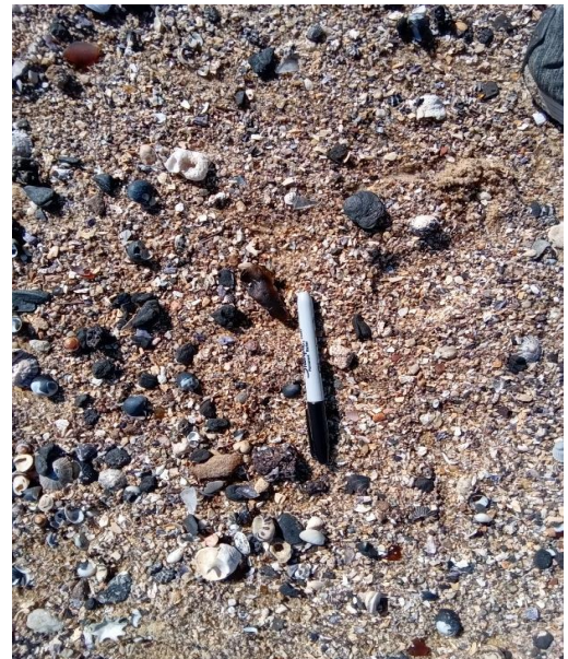
Notes: Visual clearance inspection following removal of suspected asbestos containing FC fragment.
