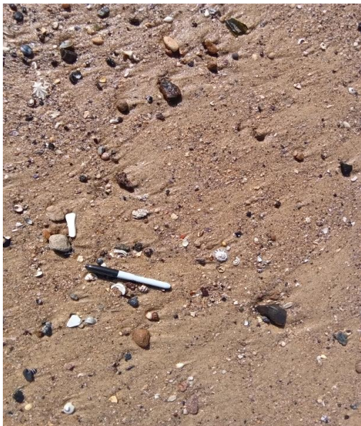
Notes: Visual clearance inspection following removal of suspected asbestos containing FC fragment.
