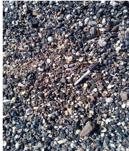
Notes: Visual clearance inspection following removal of suspected asbestos containing FC fragment.
