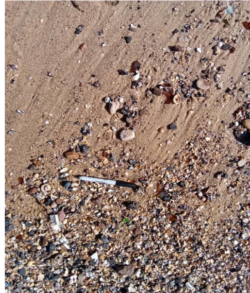
Notes: Visual clearance inspection following removal of suspected asbestos containing FC fragment.
