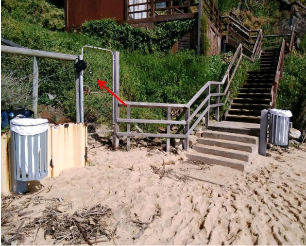
Location: Western elevation, Beach entry, on fence Result: 0 fibres / 100 fields Image Id: 230215-100459
