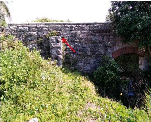
Location: Northern elevation, on stone retaining wall Result: <0.01 f/ml Image Id: 230215-101324
