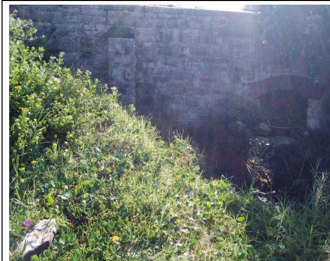
Location: Northern elevation, on stone retaining wall Result: <0.01 f/ml Image Id: 230506-083909
