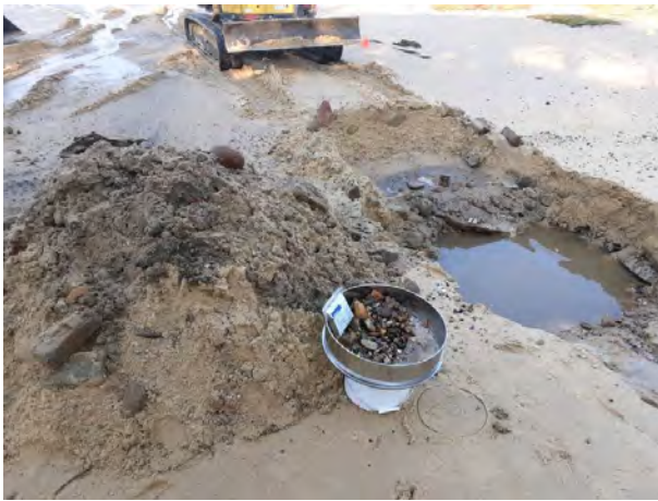
Middle beach, TP22_1.0, Fill with brick, glass, tile and concrete under top sand.
