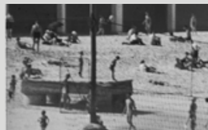
The concrete columns of the first shark tower, 1937 State Library of NSW .
