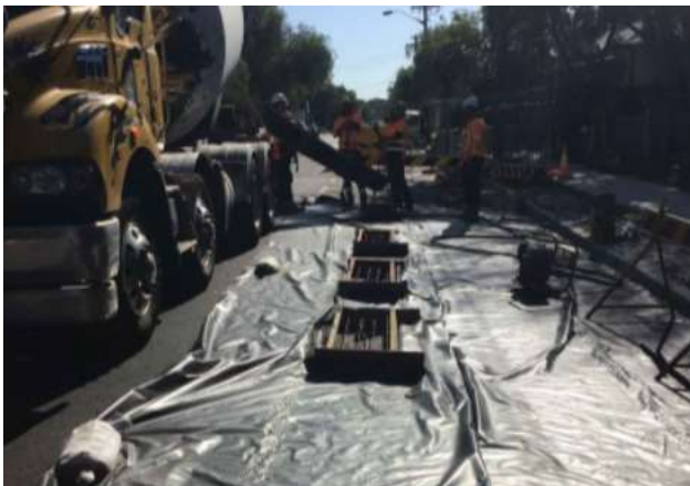
Formwork for concrete kerb separators for cycleway – Doncaster Avenue, facing north
