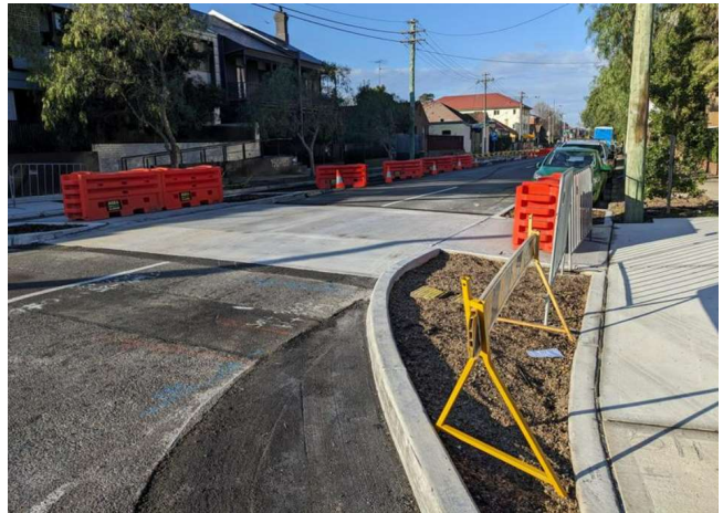
Raised pedestrian crossing - Doncaster Avenue at Darling Street, facing southeast
