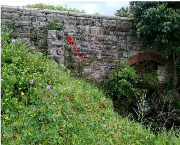
Location: Northern elevation, on stone retaining wall Result: <0.01 f/ml Image Id: 230512-102235
