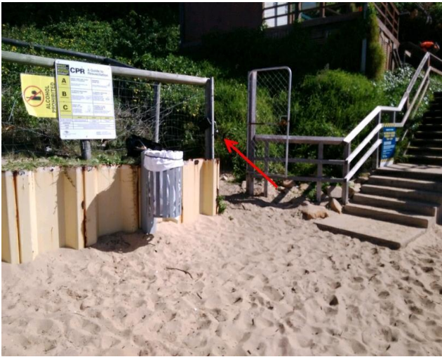
Location: Western elevation, Beach entry, on fence Result: <0.01 f/ml Image Id: 230512-102215
