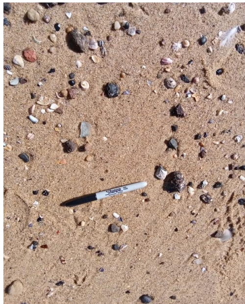
Notes: Visual clearance inspection following removal of suspected asbestos containing FC fragment.
