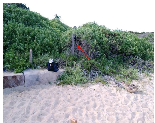
Location: Southern elevation, on pole Result: <0.01 f/ml Image Id: 221229-130615
