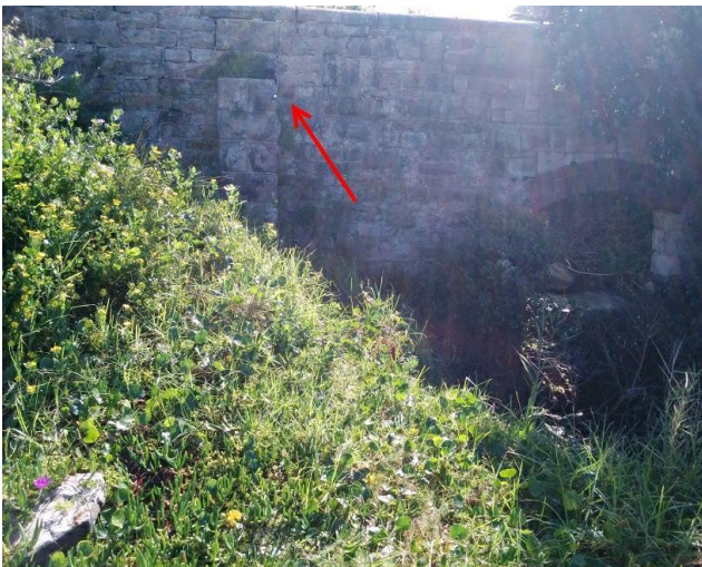
Location: Northern elevation, on stone retaining wall Result: <0.01 f/ml Image Id: 230603-122113
