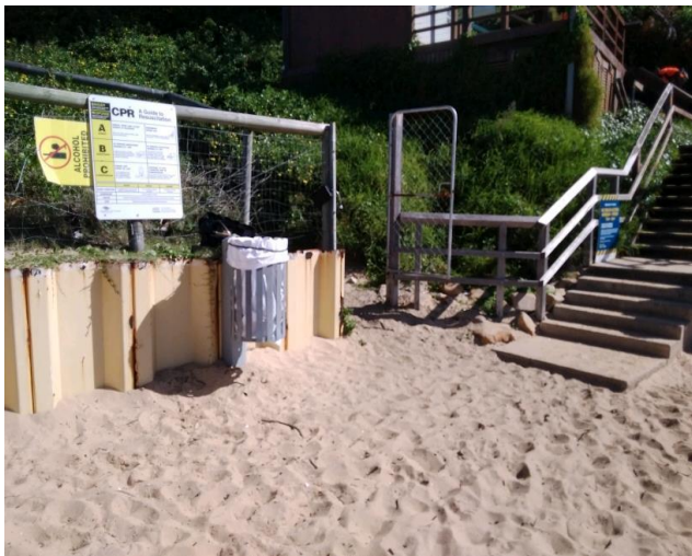
Location: Western elevation, Beach entry, on fence Result: <0.01 f/ml Image Id: 230504-125832
