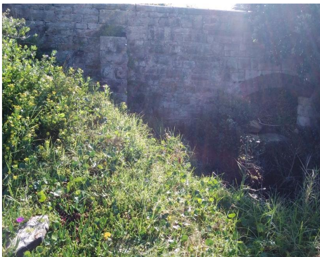
Location: Northern elevation, on stone retaining wall Result: <0.01 f/ml Image Id: 230504-125846
