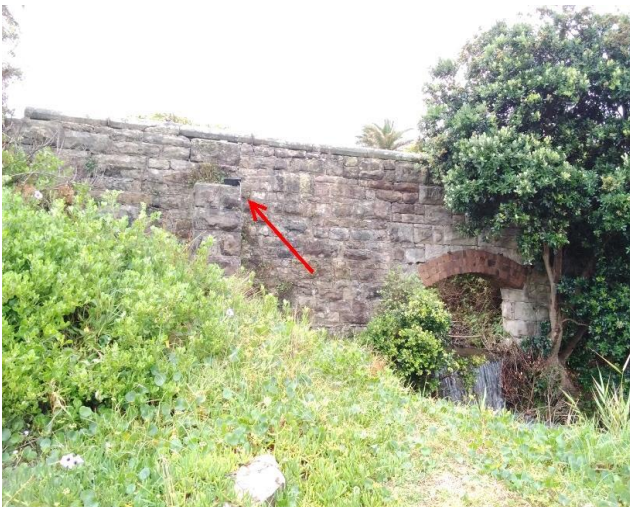
Location: Northern elevation, on stone retaining wall Result: <0.01 f/ml Image Id: 230303-094815
