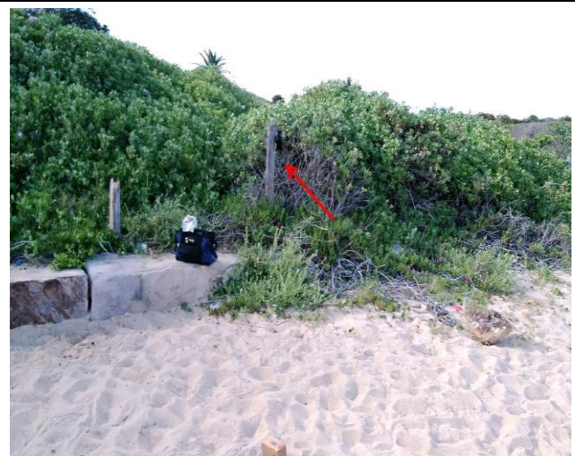
Location: Southern elevation, on pole Result: <0.01 f/ml Image Id: 230120-114826
