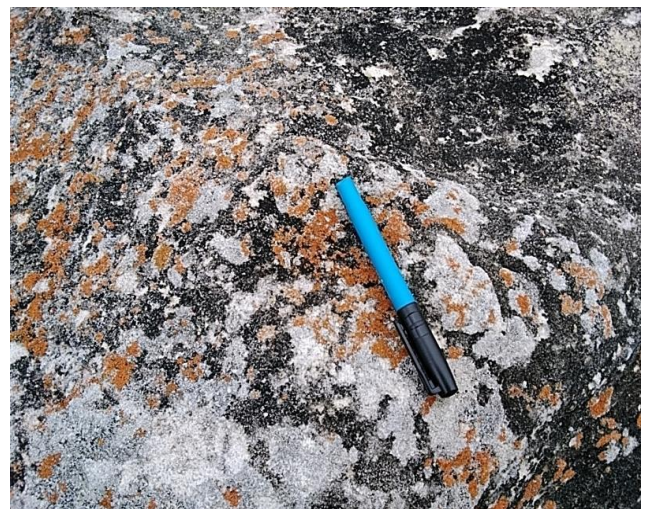
Notes: Visual inspection of removal item following removal
