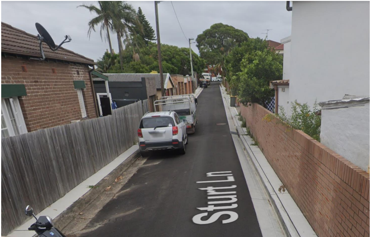
Photo 13: Sag point in Sturt Lane, showing new kerb/guttering and inlets
