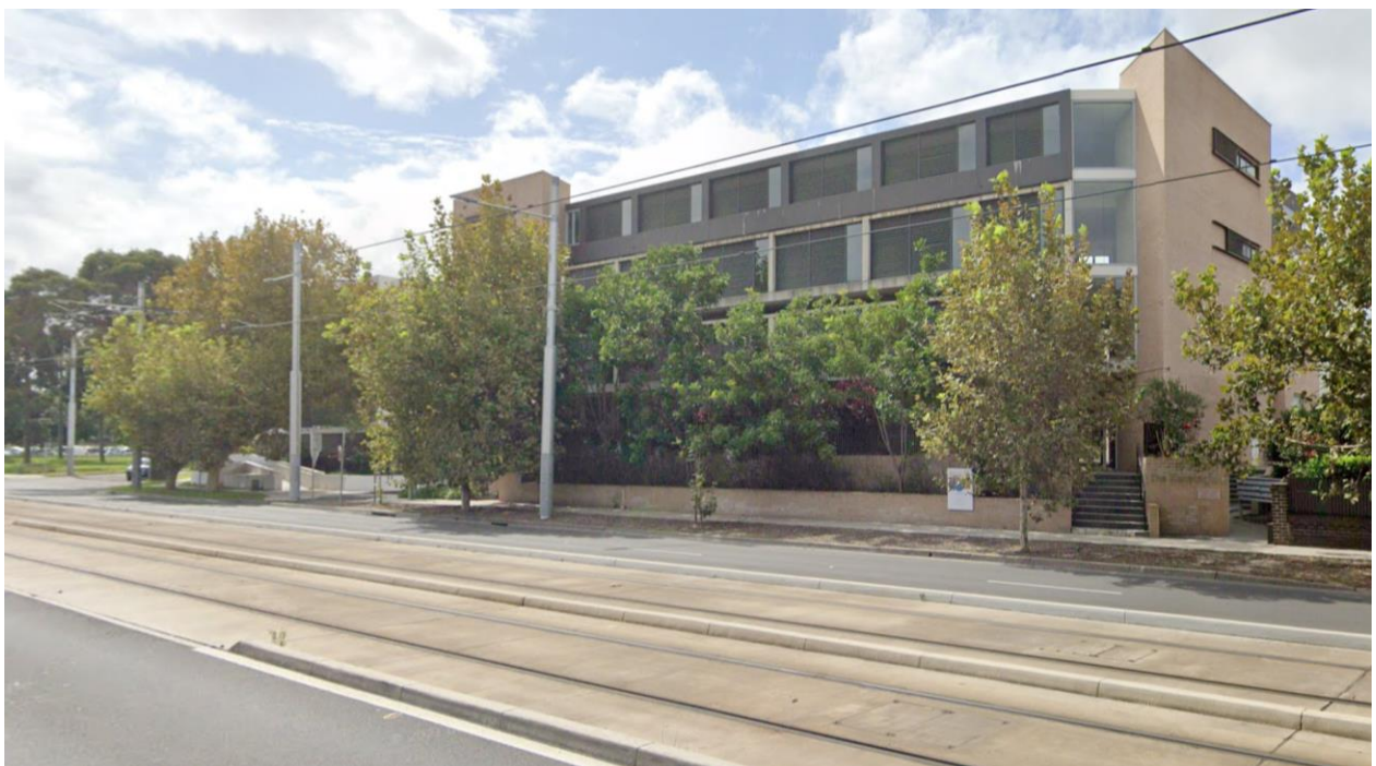
Photo 4: Raised development at 10-20 Anzac Parade adjacent to Tay Lane sag point
