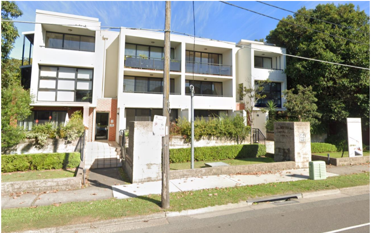
Photo 3: Raised development at 17-19 Alison Road adjacent to sag point
