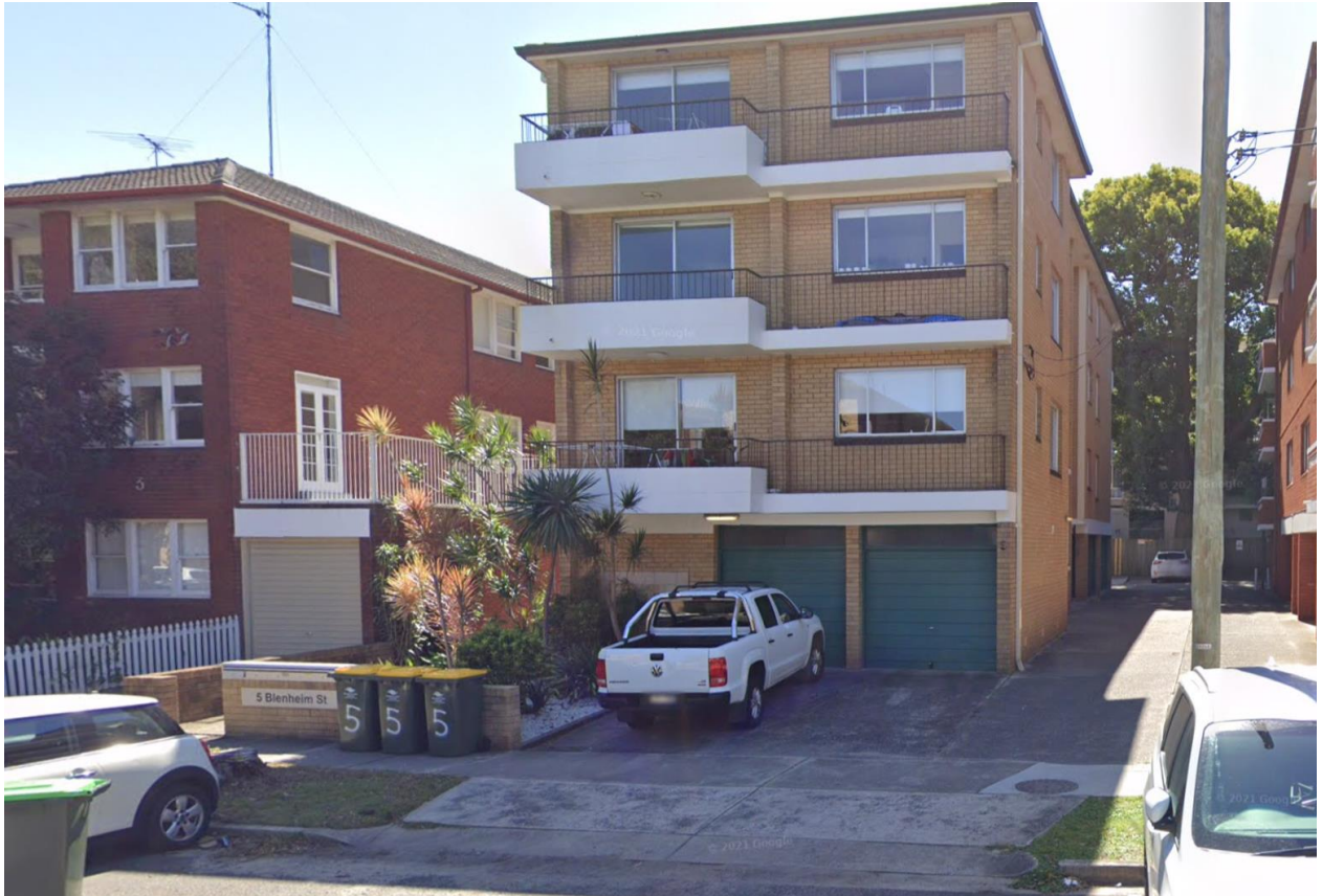
Photo 7: Existing overland flow path from sag point at 5 Blenheim Street (looking upstream)
