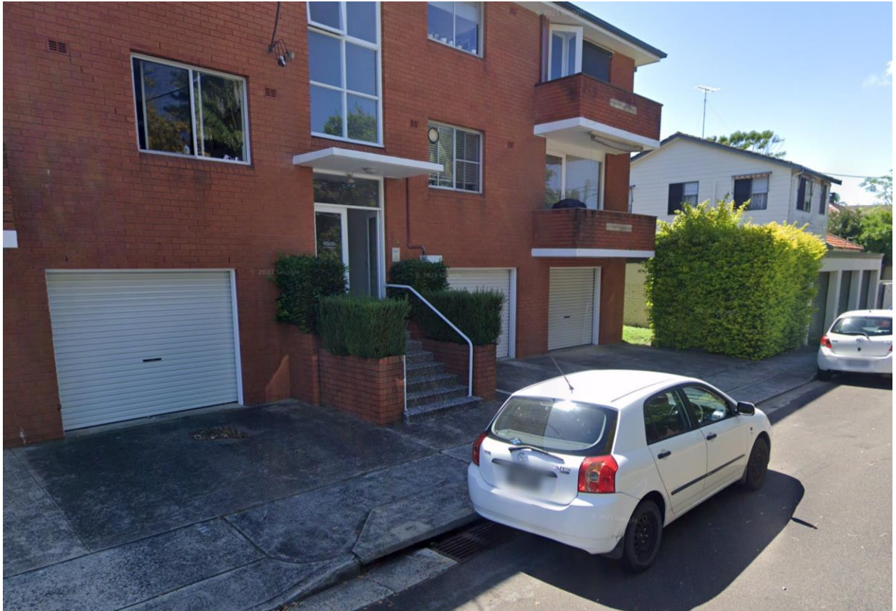
Photo 11: Elevated existing development adjacent to Jacques Street sag point
