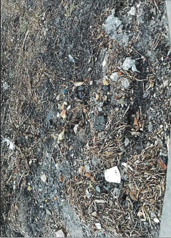
FILL EMBANKMENT & ASBESTOS, MILITARY ROAD ENTRY
