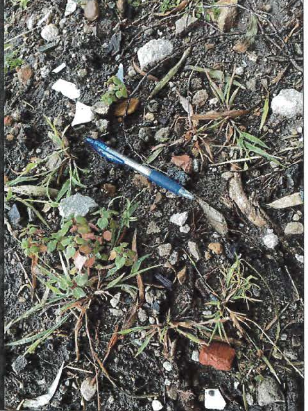
BONDED ACM IN SOIL PILE, WEST, PRINCE OF WALES DR
