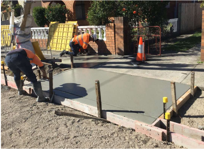
New residential driveway - Doncaster Avenue, north for Koorinda Avenue, facing east
