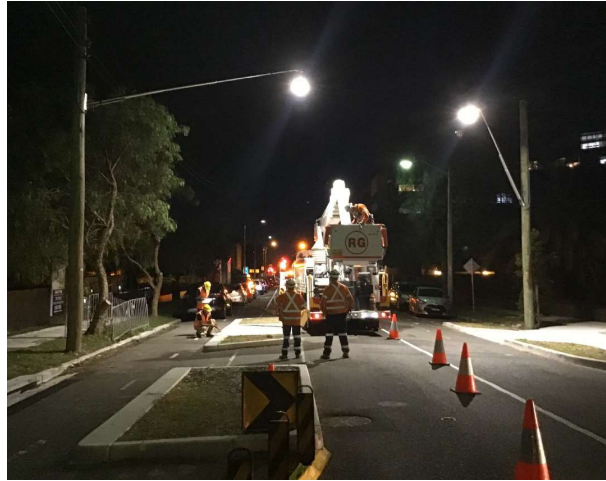
Lighting works - Doncaster Avenue at Darling Street, facing south
