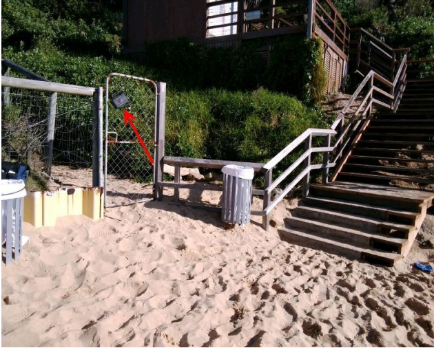
Location: Western elevation, Beach entry, on fence Result: <0.01 f/ml Image Id: 230624-100034
