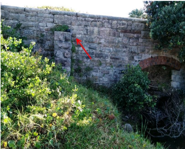
Location: Northern elevation, on stone retaining wall Result: <0.01 f/ml Image Id: 230624-100736
