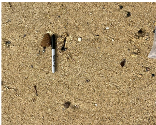
Notes: Visual clearance inspection following removal of asbestos containing FC Sheeting fragment.
