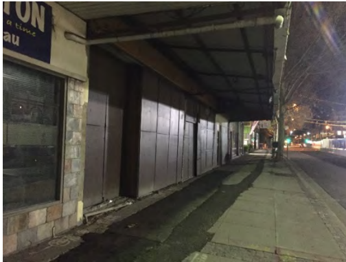
Figure 102: Vacant shop fronts Anzac Parade, Kensington Source: Randwick City Council
