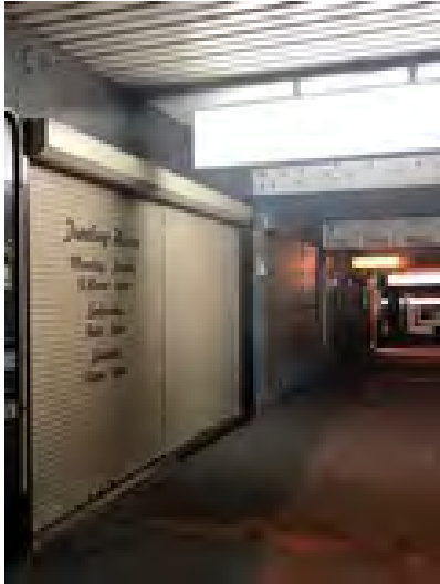
Figure 45: Matraville town centre looking north Bunnerong Rd. Presence of closed businesses and roller shutters presents an unwelcoming environment with minimal pedestrian activity.
