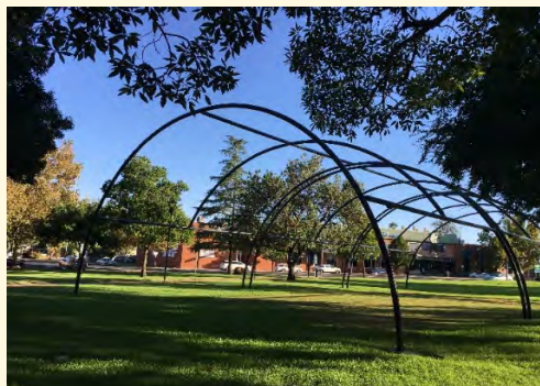
Figure 79: Multifunctional adaptable structure for events, Cooke Park, Parkes NSW Source: Randwick City Council
