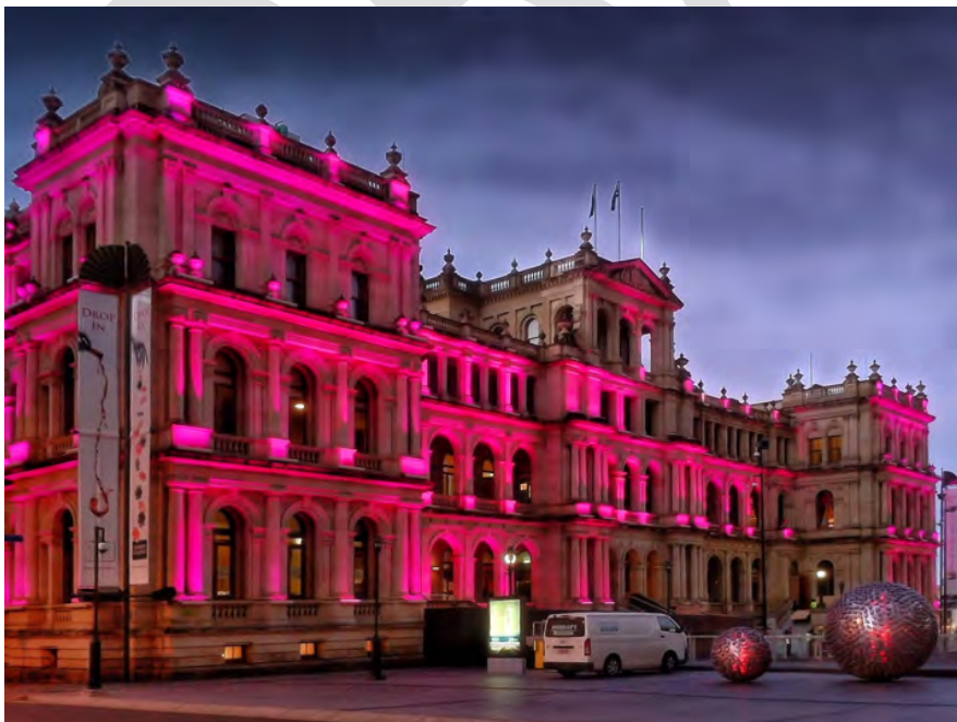
Figure 94: Example of temporary landmark lighting
