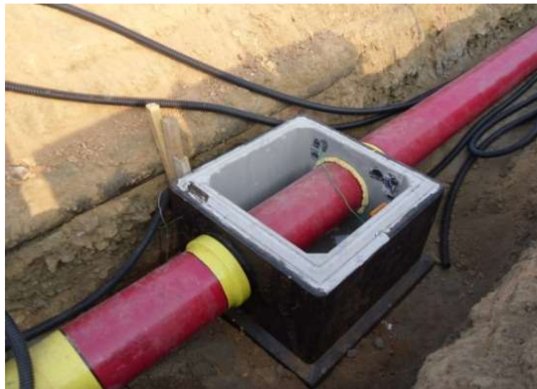
Figure 3-9 - Installed Pipework Showing Cabling for Electric and Compressed Gas
