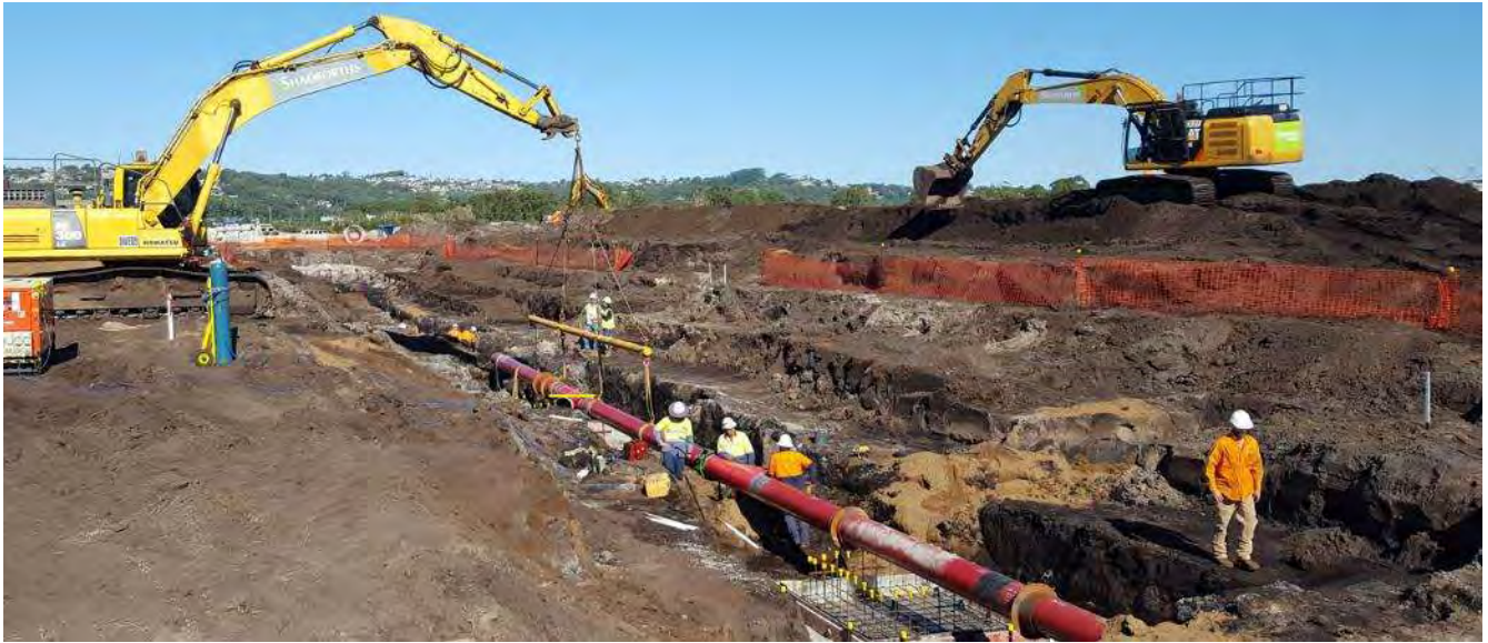
Figure 3-13 - AWCS Pipe Installation in Maroochydore City
