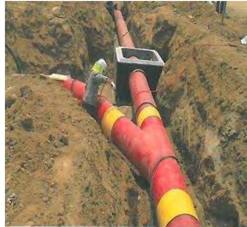
Figure 3-8 - Photographs Showing Installed Pipe Bends and Branch Connections
