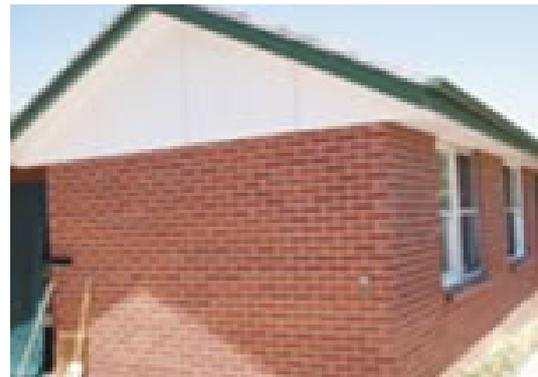
Fig 2: Asbestos cement sheeting under eaves & gables
