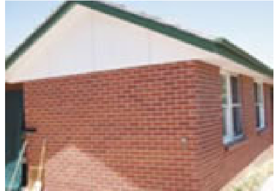
Fig 2: Asbestos cement sheeting under eaves & gables
